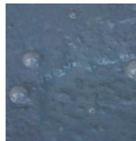
**INSPECTION** After application of the primer inspect the surface to ensure that it is completely covered with a film of epoxy. Occasionally concrete can be extremely porous and air will escape through successive coats of epoxy causing bubbles or craters in the surface of finishing coats.
