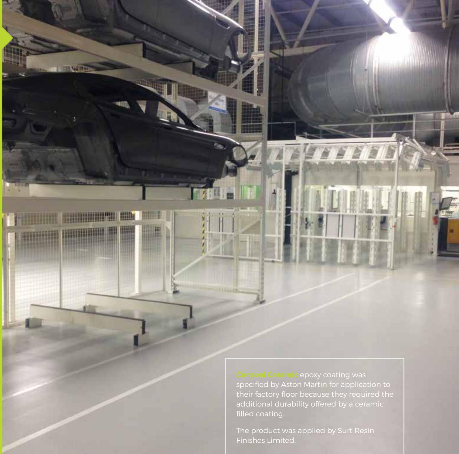
**Conseal Ceramic** epoxy coating was specified by Aston Martin for application to their factory floor because they required the additional durability offered by a ceramic filled coating.
