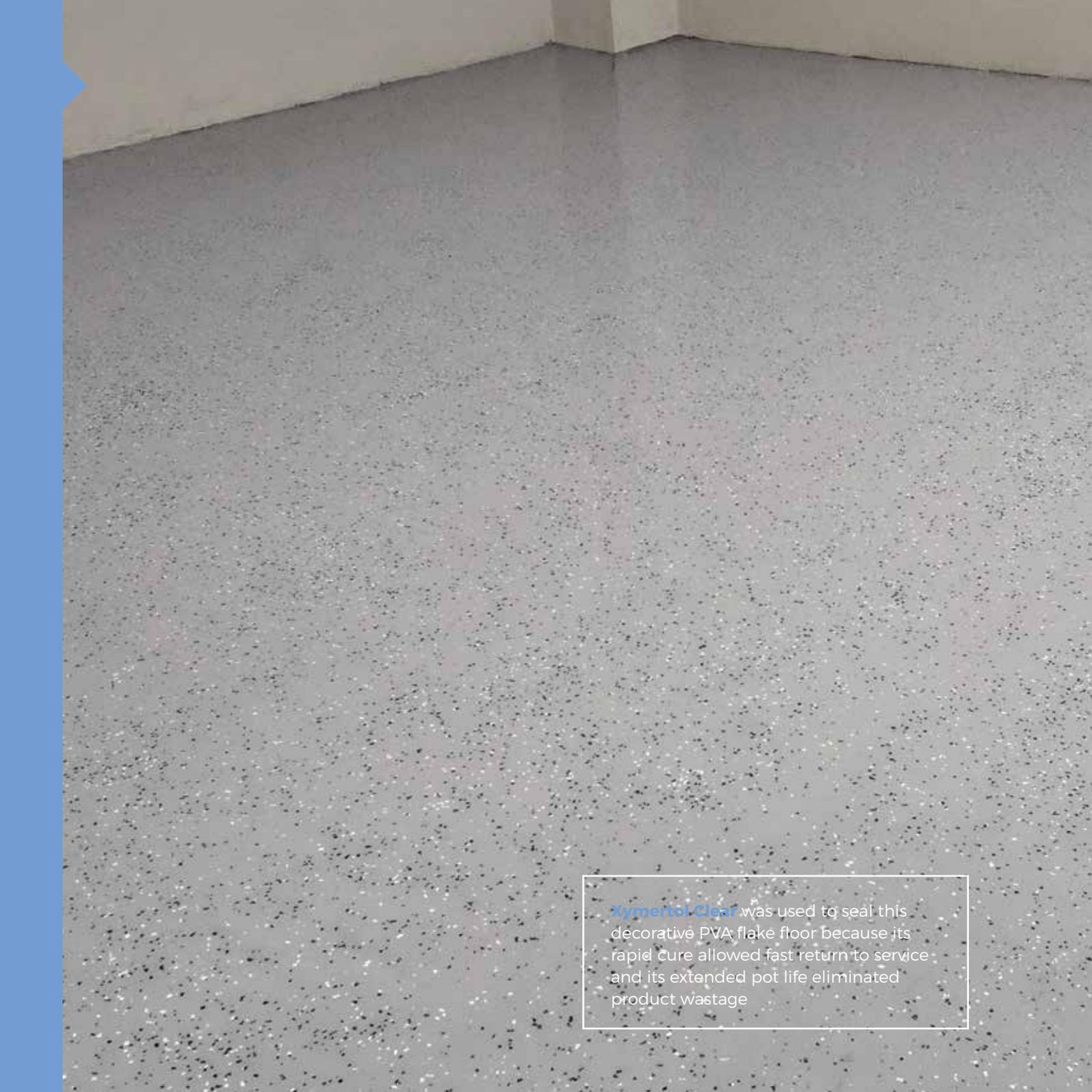
**Xymertol Clear** was used to seal this decorative PVA flake floor because its rapid cure allowed fast return to service and its extended pot life eliminated product wastage
